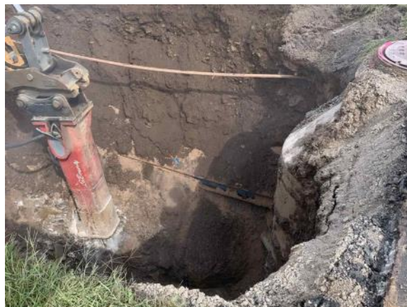
Excavation to expose and tie into existing sanitary sewer manhole (8/31/2021)
