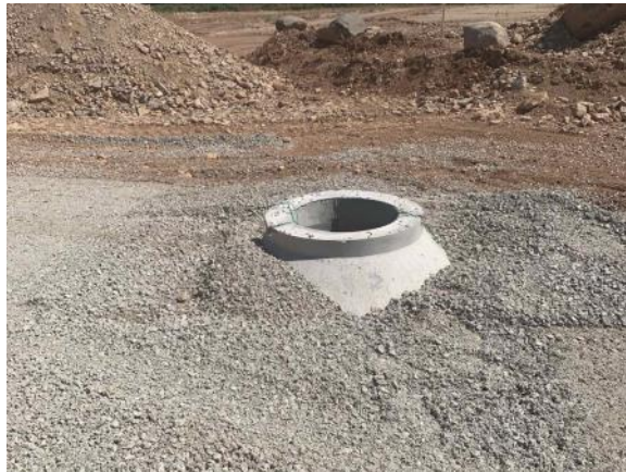
Completed manhole #11 near school main entrance (8/17/2021)
