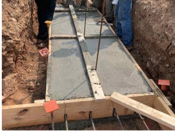
Concrete footing with rebar reinforcement (8/26/2021)
