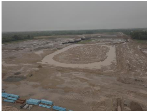
Aerial view of future football field and track (8/27/2021)
