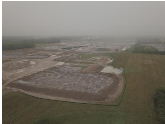
Aerial view of future baseball/softball fields (8/27/2021)
