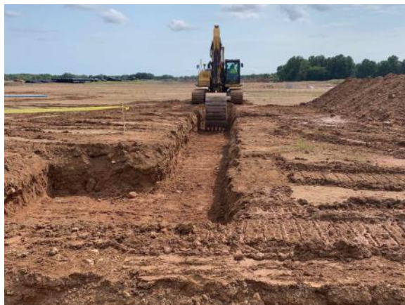
Excavation for concrete footings and foundations (8/25/2021)
