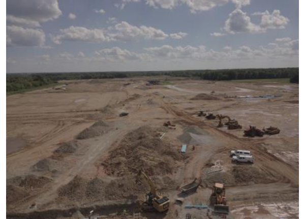
Aerial view of project looking South (8/30/2021)
