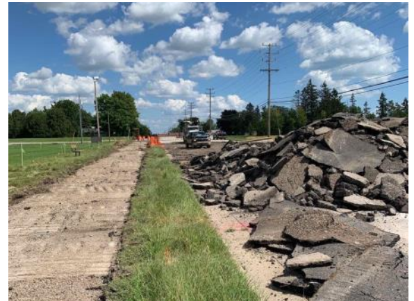
Asphalt starts to be removed in County Hwy II (8/30/2021)
