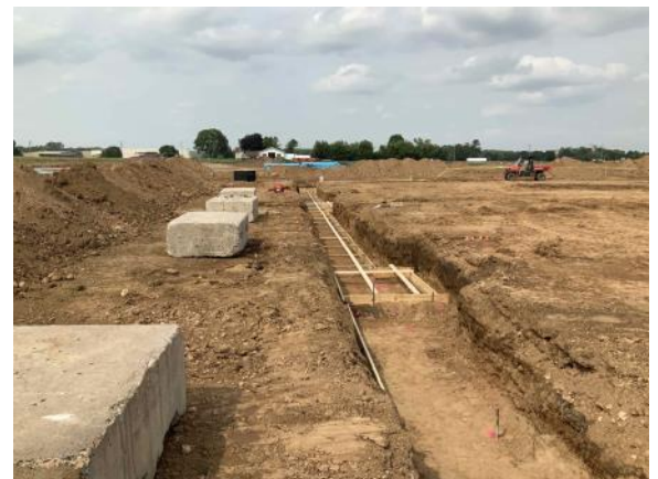
Formwork begins for concrete footings (8/26/2021)
