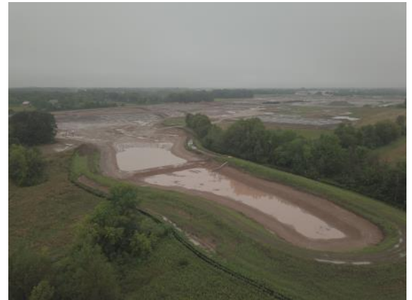
Aerial view of retention pond (8/27/2021)
