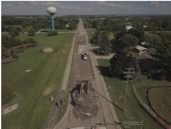
Aerial view of County Hwy II roadwork looking East (8/30/2021)
