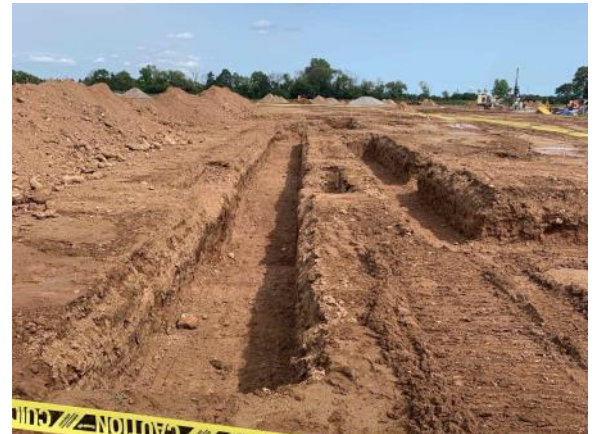
Excavation for concrete footings and foundations (8/25/2021)
