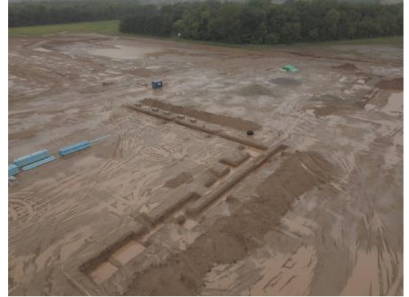
Aerial view of footing excavation in the future gym (8/27/2021)
