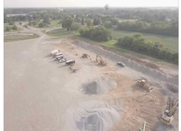
Sanitary sewer installation in NE corner of site (8/5/2021)
